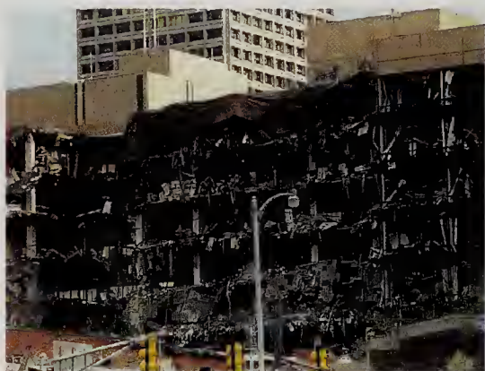
The north side of the Alfred P. Murrah building lies in ruins following the explosion of a home-made bomb.
